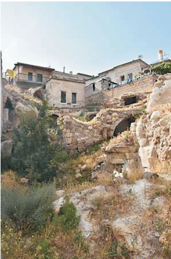
Buildings on all of the hills
