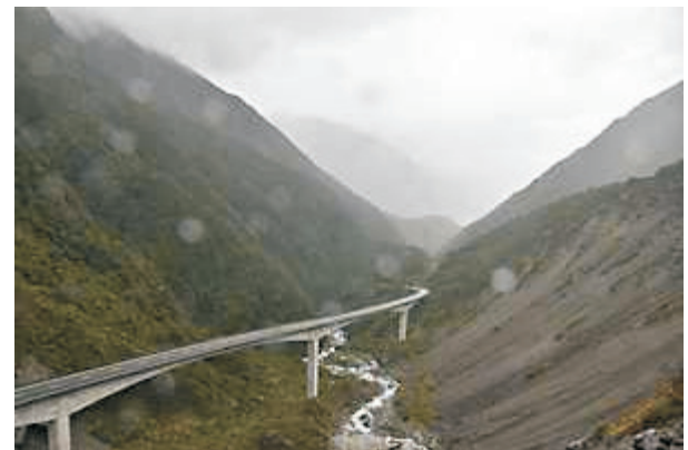
The drizzle arrived over the new viaduct
