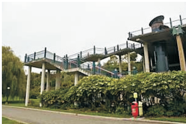
Back up the steps to the road
