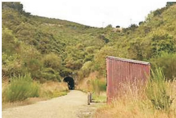
Gangers hut with tunnel in the background
