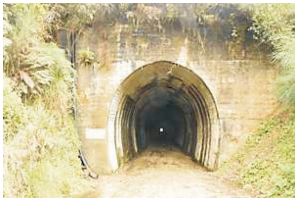
The tunnel was in good order ...
