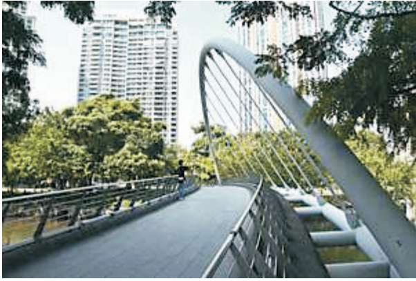
Jiak Kim Bridge - as previously discussed
