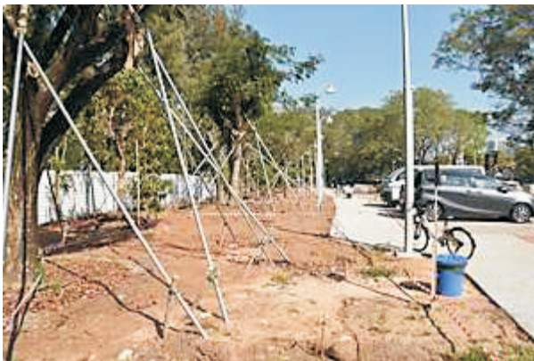
Lots of work going on
