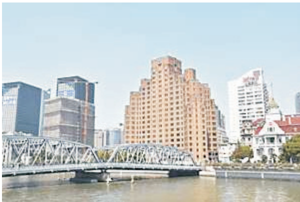
The Waibaidu Bridge & the Broadway Hotel
