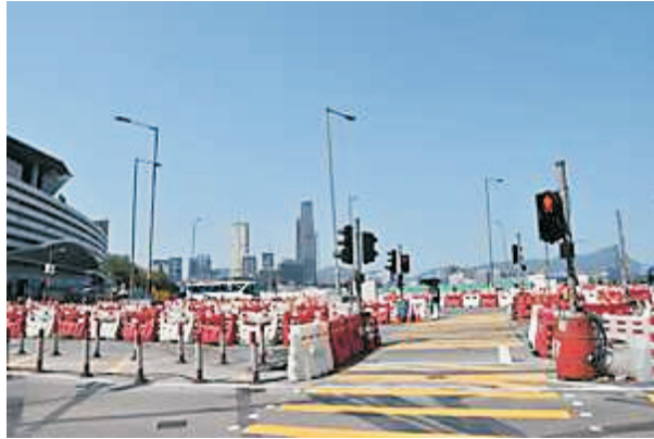
Construction work everywhere
