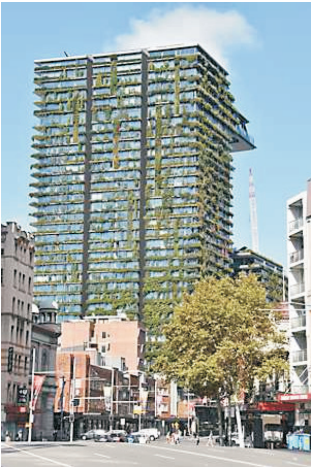
A very green building
