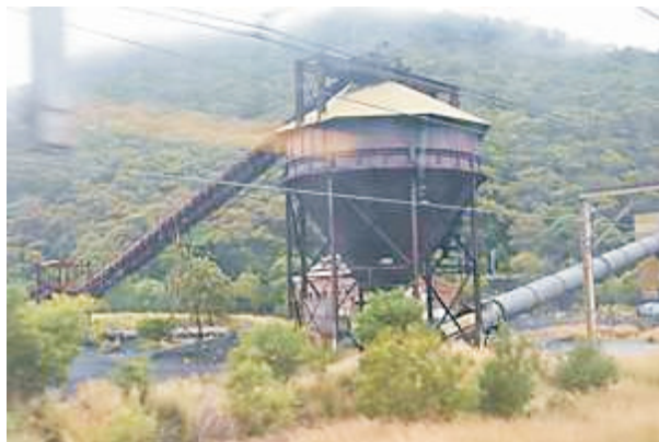
Past some strange industrial buildings
