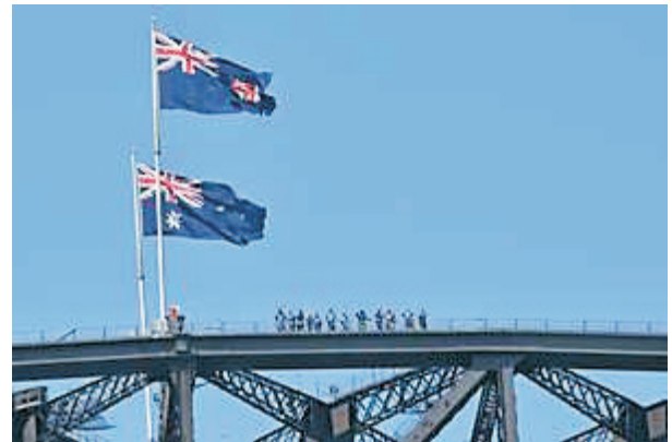
Under the bridge walkers
